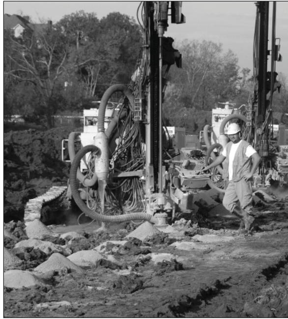
An operator drills holes for a trench line blast for installation of a sewer line in Madison County.
